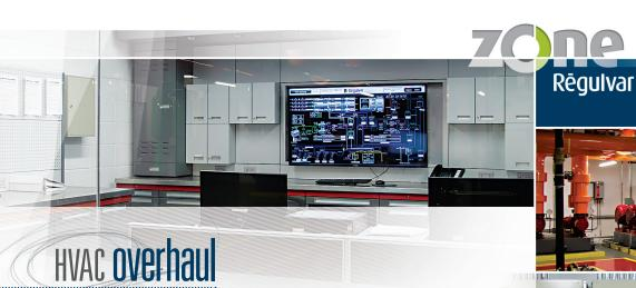
The building automation system installed by Regulvar controls the HVAC systems on all floors. In total, the system has over 5,000 control points a number that continues to grow as renovations are completed.
